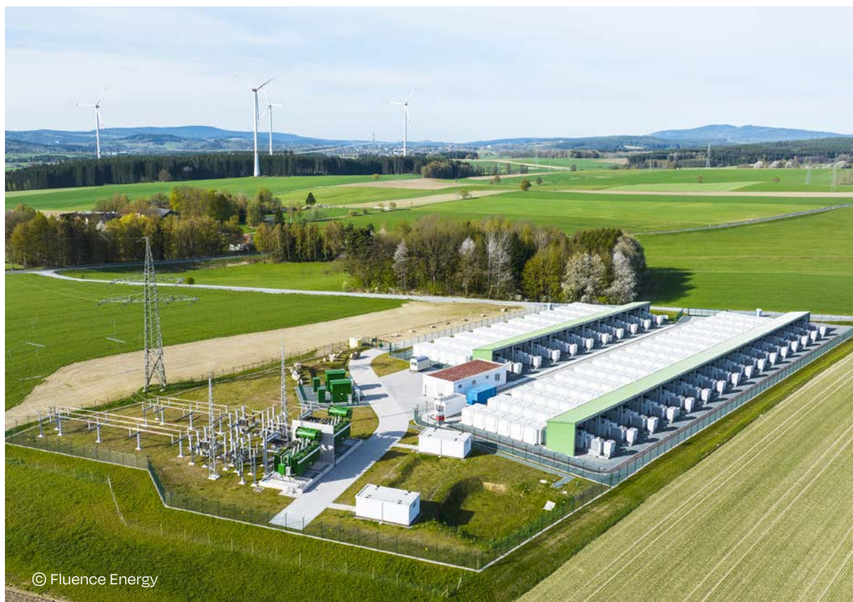
Arzberg Battery Storage Project, Arzberg, Bavaria, Germany — 100 MW / 200 MWh battery energy storage system
