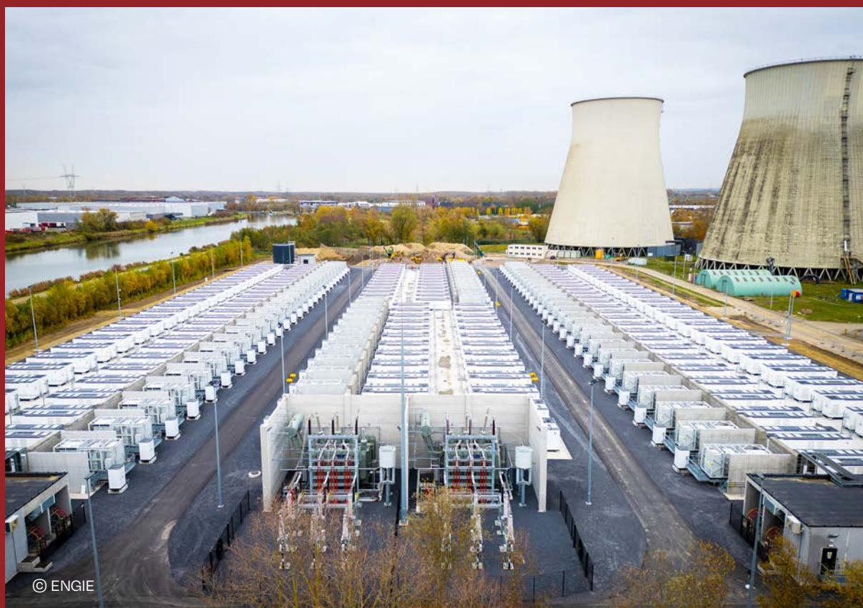
BESS Vilvoorde, Vilvoorde, Belgium — ENGIE's 200 MW / 800 MWh battery park, among the largest in Europe
