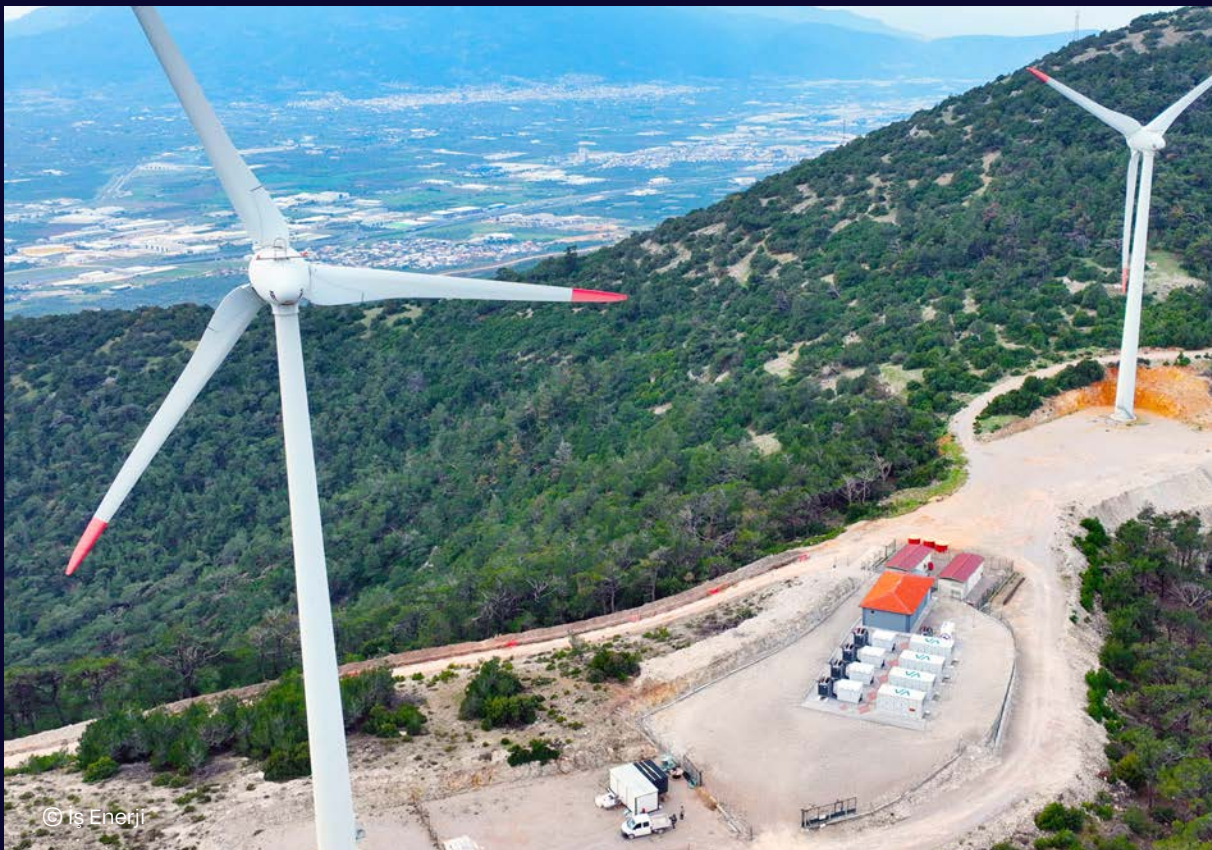
Ege RES, Kemalpaşa, İzmir, Türkiye — 12.8 MWe / 15.17 MWh battery energy storage system
